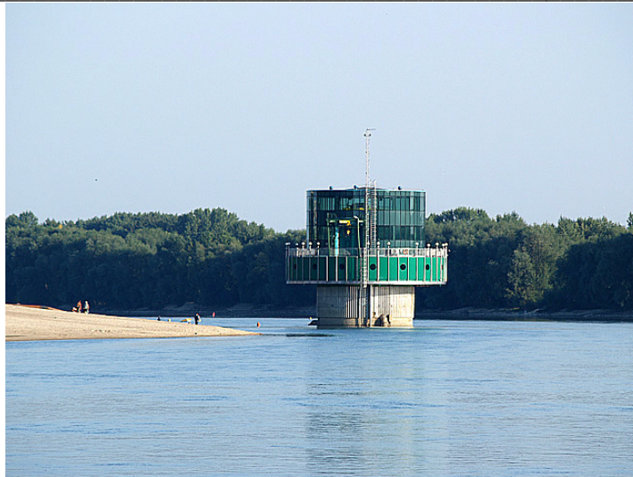
Fig. 4. Drainage systems shall also apply to installing them radially beneath the river (eg wells, "Thick Kaska" aqueduct Warsaw - Department of aqueduct Prague), and receiving water from the drains by gravity takes place in a centrally located shaft wells. 15
