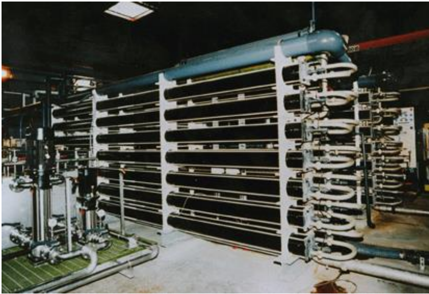
Nanofiltration water cleaning serving Mery-sur-Oise, a suburb of Paris, France
