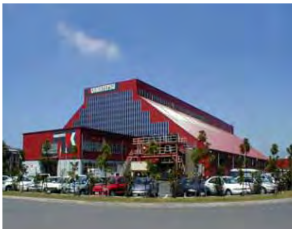
Photo 2. MSW gasification plant in Chiba (Japan)
