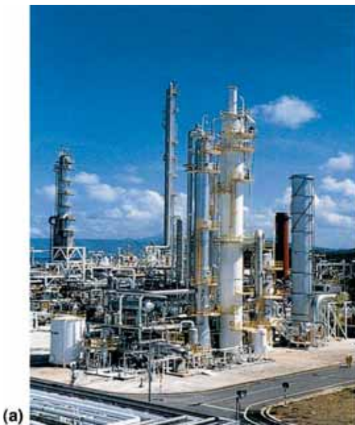
Figure TS.4. (a) CO 2 post-combustion capture at a plant in Malaysia. This plant employs a chemical absorption process to separate 0.2 MtCO 2 per year from the flue gas stream of a gas-fired power plant for urea production (Courtesy of Mitsubishi Heavy Industries). (b) CO 2 pre-combustion capture at a coal gasification plant in North Dakota, USA. This plant employs a physical solvent process to separate 3.3 MtCO 2 per year from a gas stream to produce synthetic natural gas. Part of the captured CO 2 is used for an EOR project in Canada.
